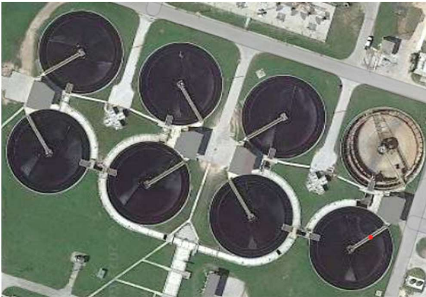
Primary Clarifier Effluent Channels
